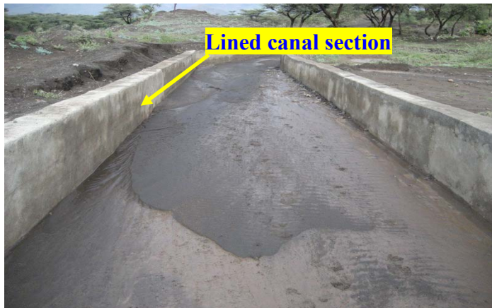
Figure 21. Picture of a lined main canal section filled with some sediment
