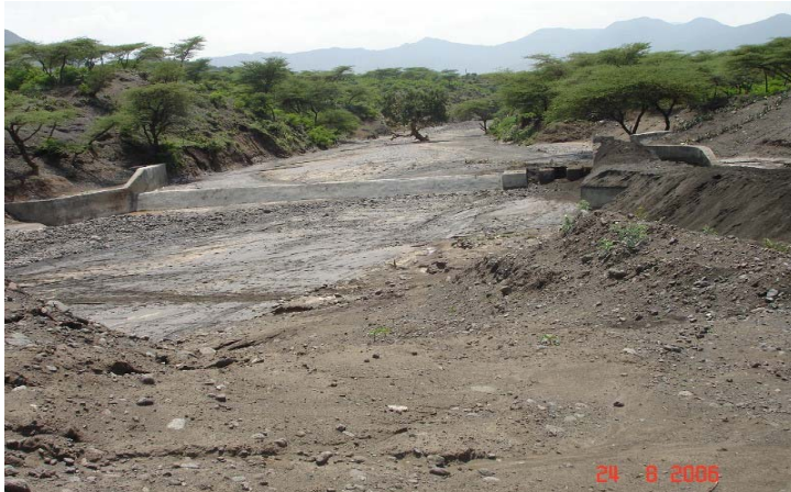
Figure 14. Fokisa spate irrigation scheme diversion headwork
