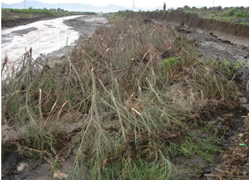
Figure 7. Traditional spate irrigation headwork in Tigray
