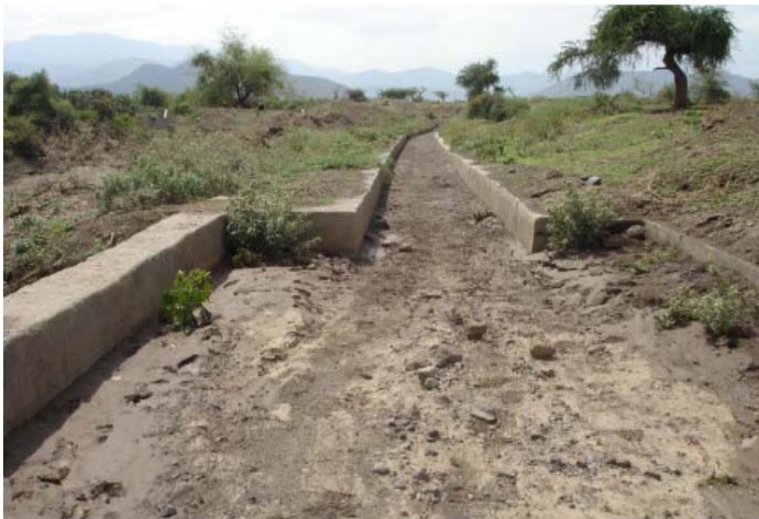
Figure 6. Sedimented canal and settling basin of spate scheme in Tigray, Ethiopia
