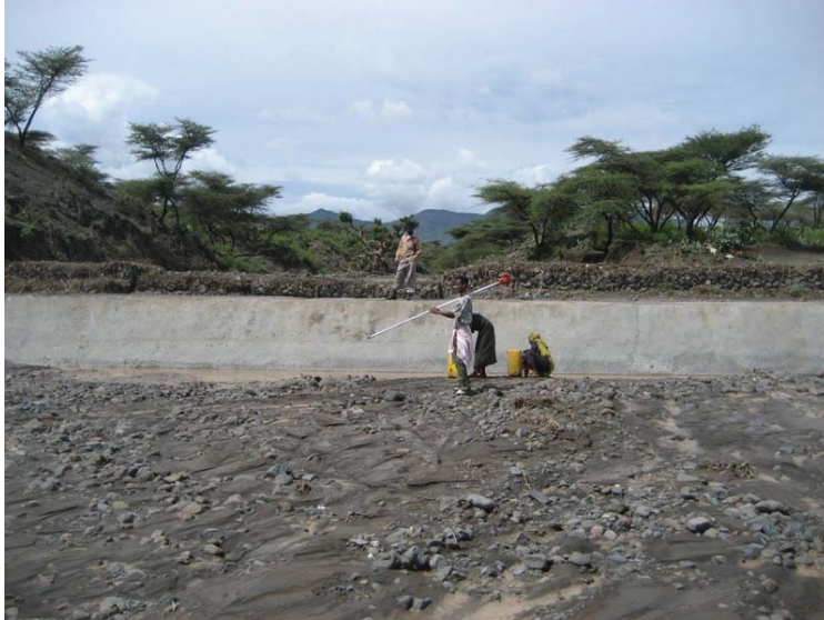
Figure 3. Gabion headwork built over the weir in Fokisa spate scheme
