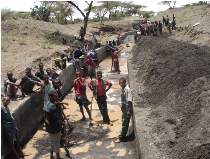
Figure 8. Farmers removing sediments from the main canal by dredging, at the Fokisa spate scheme
